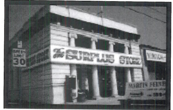
Inappropriate: Sign overpowers & ignores architectural columns.
